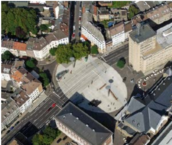
Figure 23: Example of public space with pedestrian crossing over major road, unified by materials and public realm treatment – Aachen Bahnhofplatz
